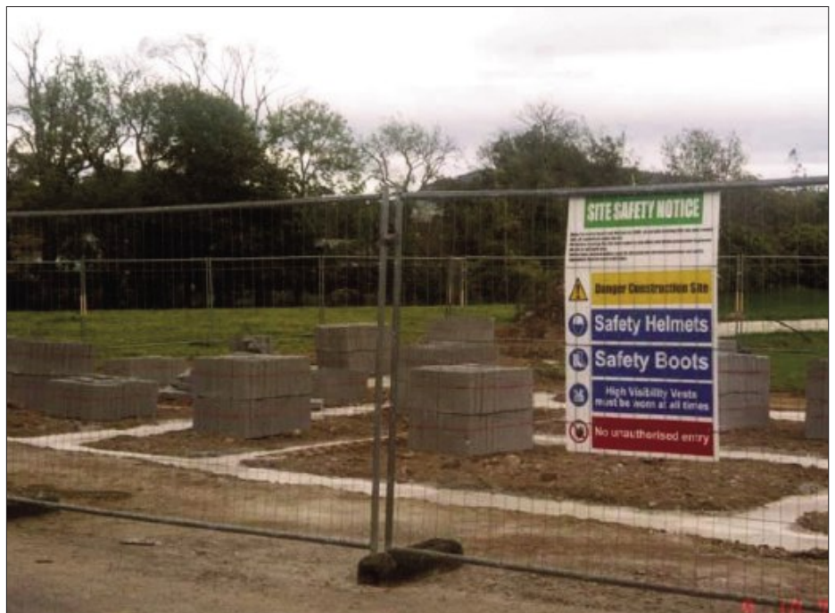
Work Under Way! Foundations of the new Club Dressing Rooms
