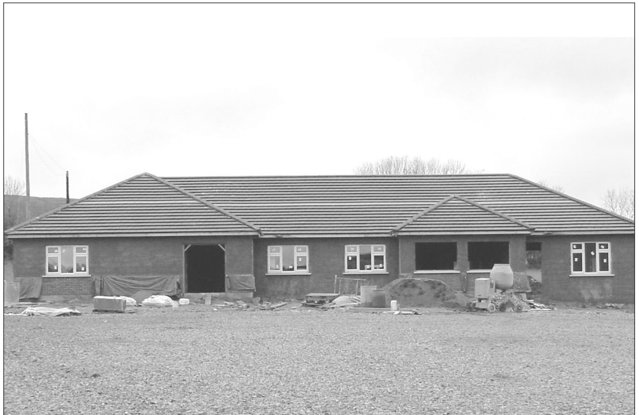
ÁRAS Ó MEALLAIGH - NEW CLUB ROOMS AT "CANON KEARNS PARK"
