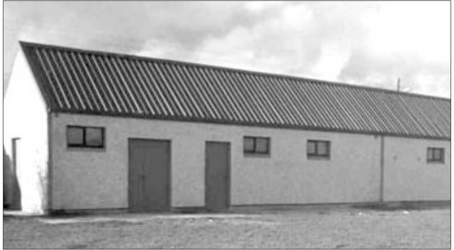
Slieverue's Refurbished Dressing Rooms
