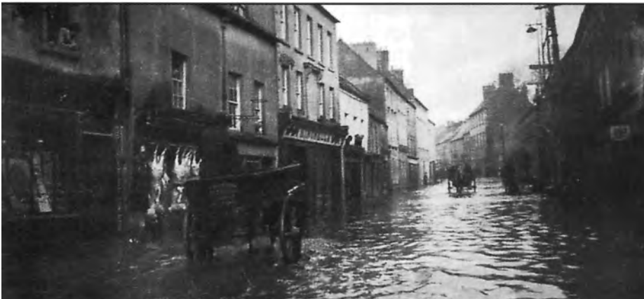
John Street flooded 1947
